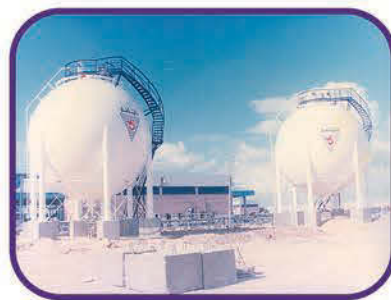
Construction of (2) L.P.G. Sphere Tanks (m3 / Tank 500) at - Damanhur/ Housh Eisa/ Behera – Delta Gas
