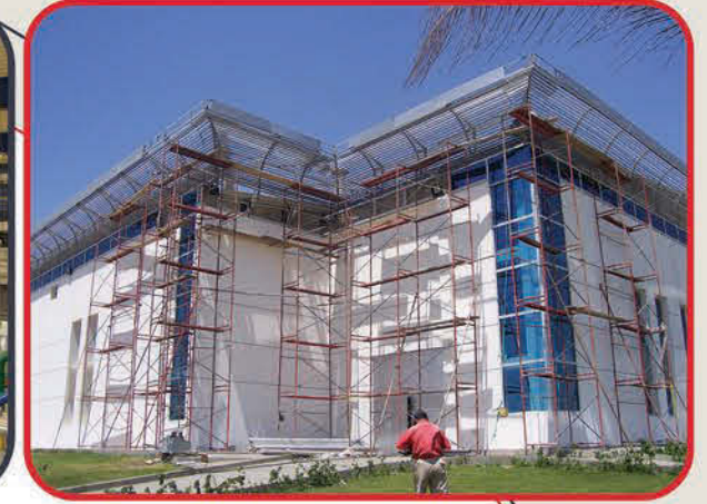
Construction Of Gas Cool Station in Smart Village
