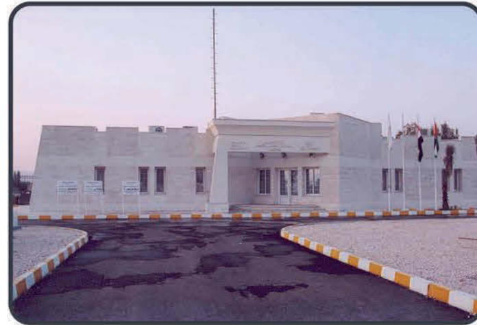
Construction Of Monitoring & Control Center – El Akaba
