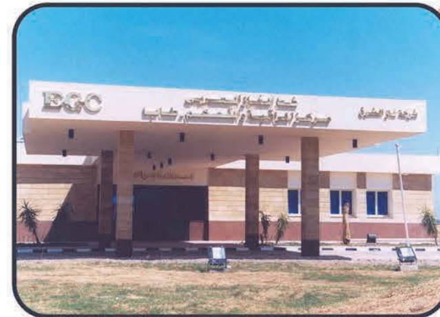
Construction Of Monitoring & Control Center – TABA
