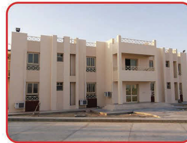
Construction Of Accommodation building in Qarun
