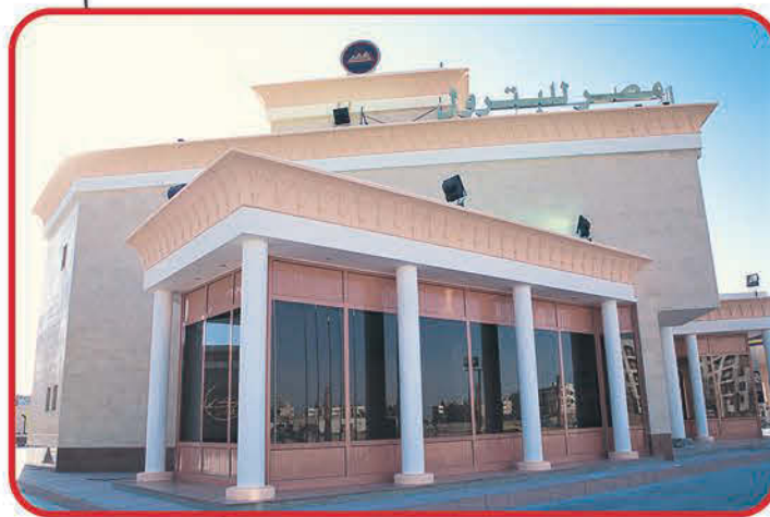
Misr Petroleum Company Construction Of Natural Gas Fueling Station
