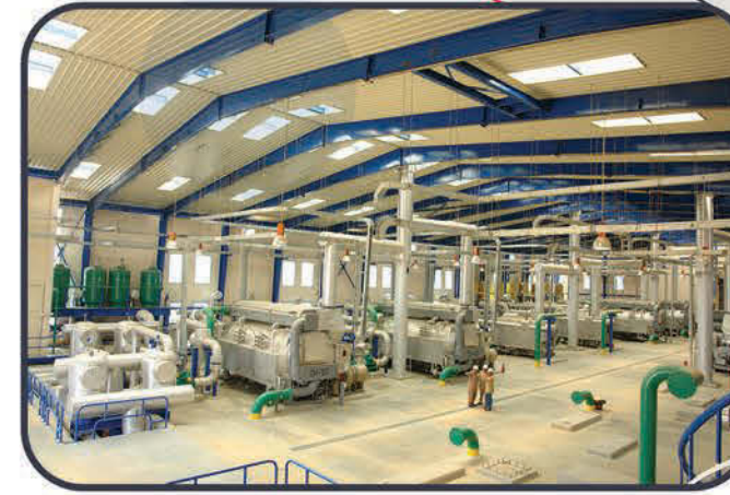
HVAC Smart Village
