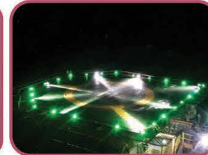
Installation Of an Integrated Explosion Proof System Of an Enhanced Lighting Fixtures System & Navigation.
