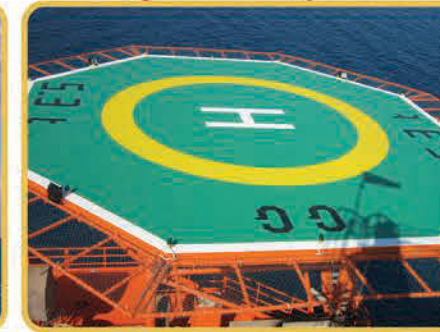
Helideck Painting, Marking and Safety Net Replacement.
