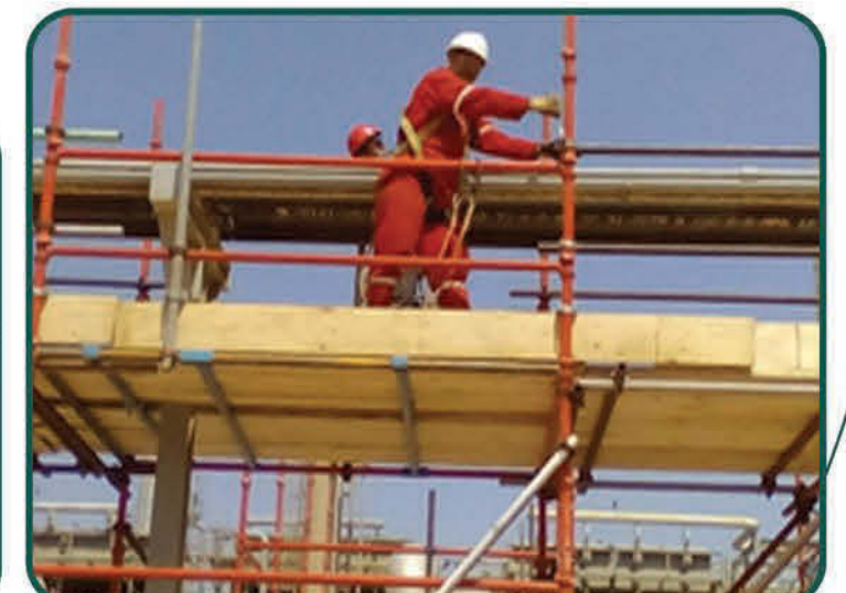
Scaffold on Gupco Ras-Shujeir
